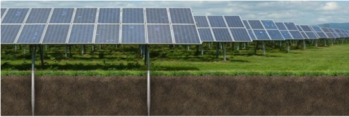
Figure 3b. Supporting Structure Overview
